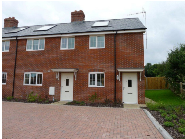
Photograph of Nos.10 (left: ground floor flat) and 11 (right: 1 st floor flat) Houghton Gardens, showing path to private gardens at rear
